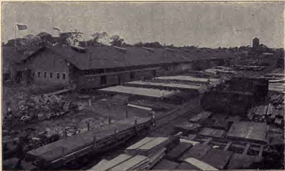
Exterior view of the I. C. C. Warehouse at Mount Hope.
