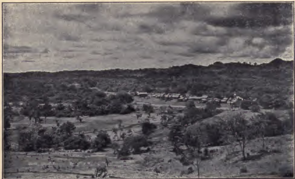
The site of the great Dam at Gatun.
