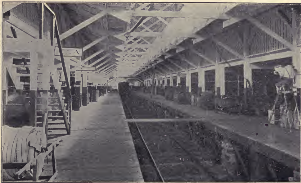
Interior view of the I. C. C. Warehouse at Mount Hope.
